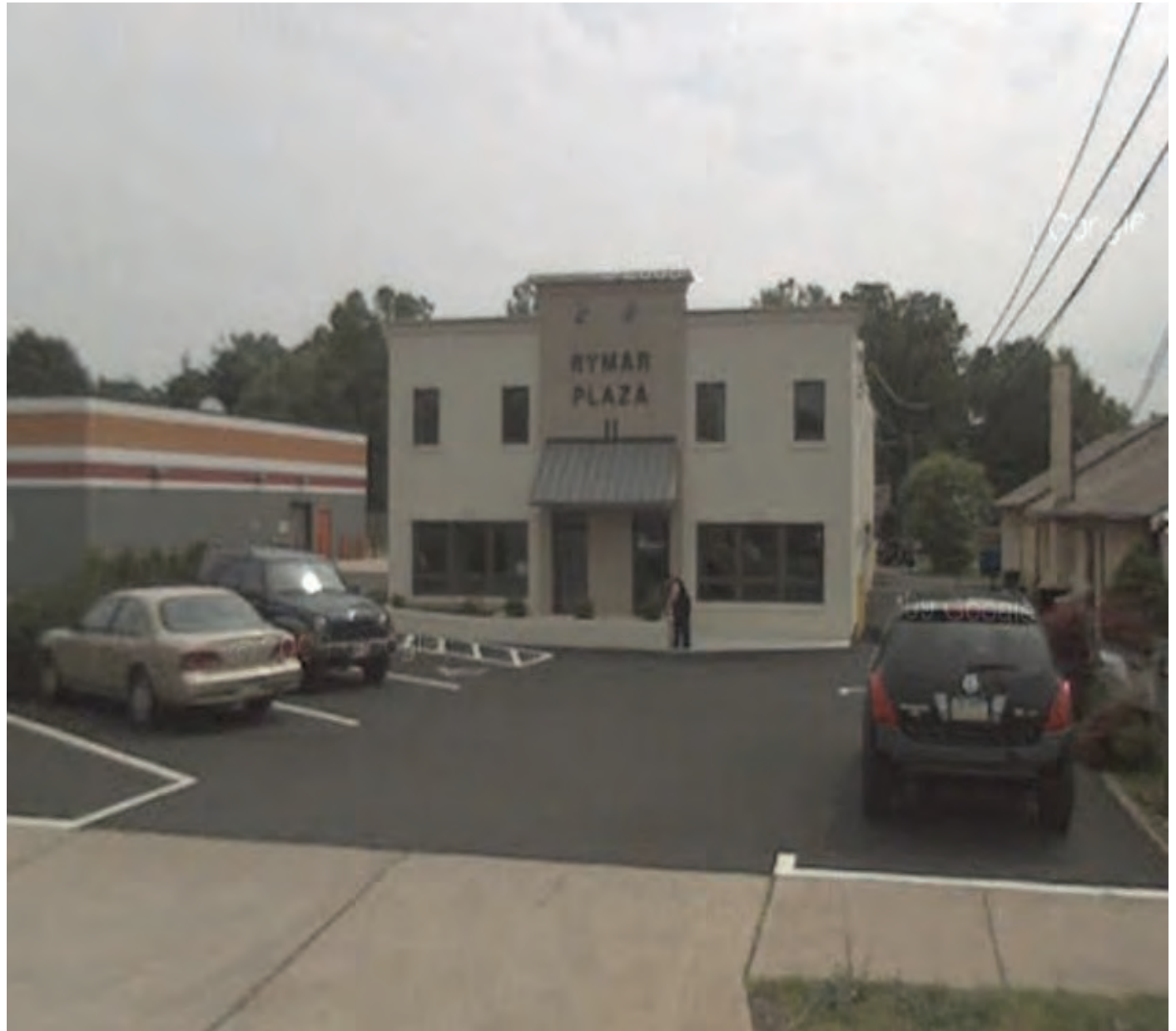
FRONT AND PARKING LOT
